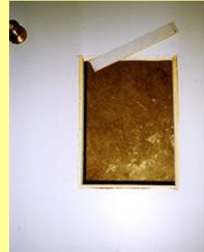
Steel door: Note hole is cut 1/2" larger to allow for 1/4" thick wood inserts. Opening 13" x 18" on the Heavy Duty Dog Door®,
