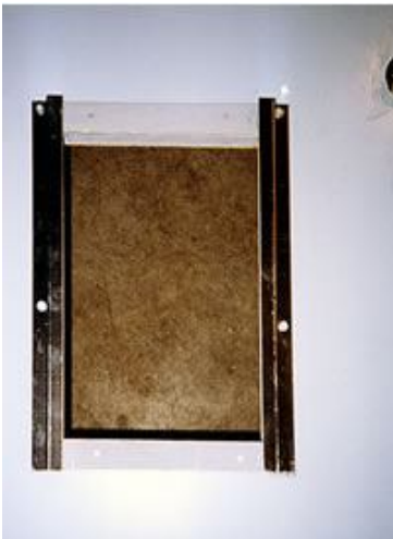
Install channel on inside of building Photo 1
