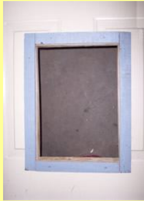
Installed door trim kit. Photo 6
